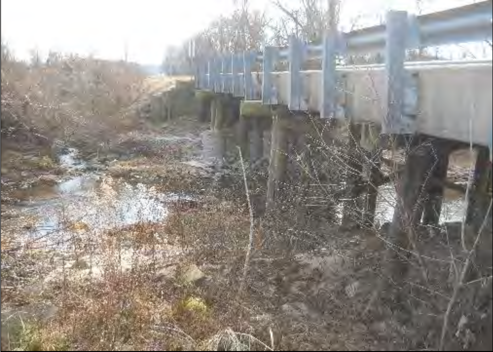
Photo 9: Upstream Profile View Of Bridge
