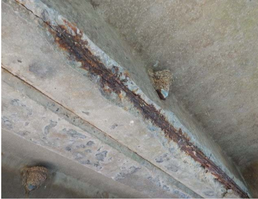
SPAN 1 SLAB "F"
