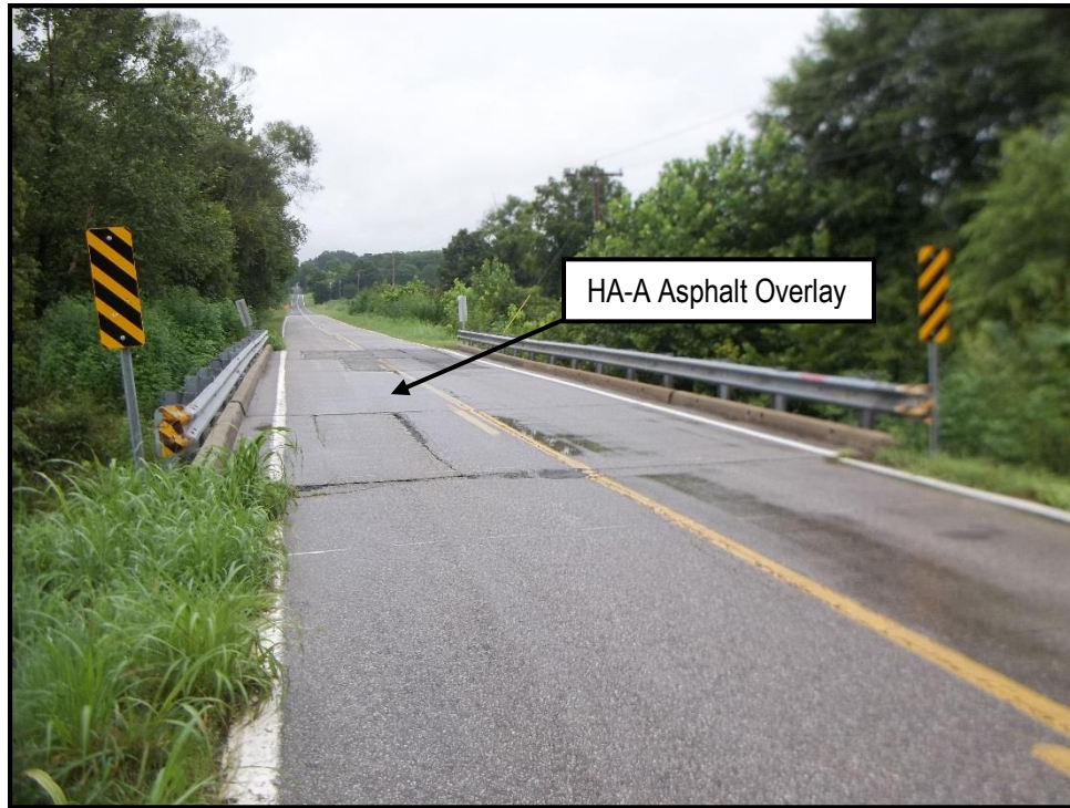
Photo 1: View of HA-A on SR-436 Bridge over Reedy Creek
