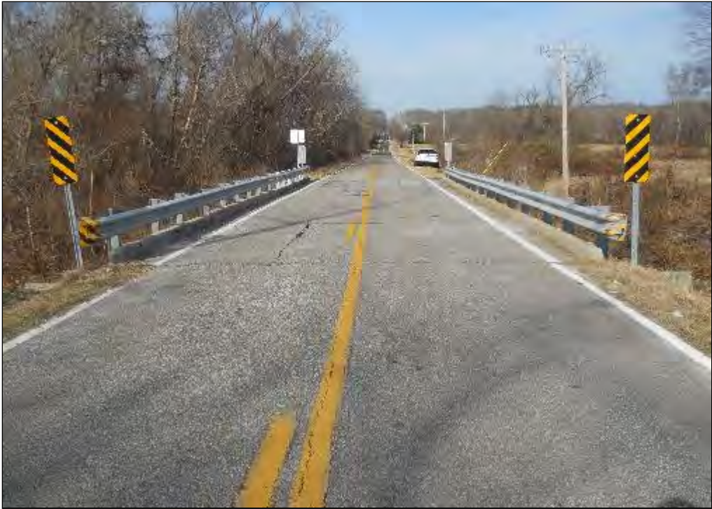
Photo 4: Northbound Bridge Approach
