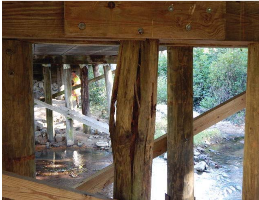
BENT 1 A PILE "C"
