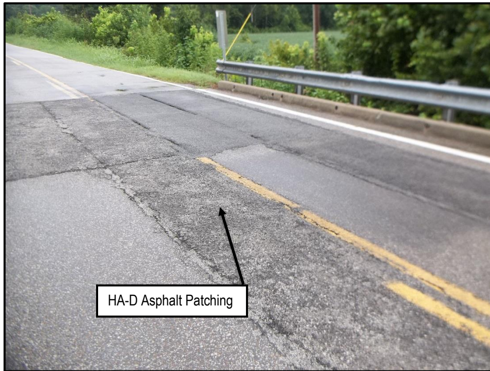
Photo 5: View of HA-D on SR-436 Bridge over Reedy Creek
