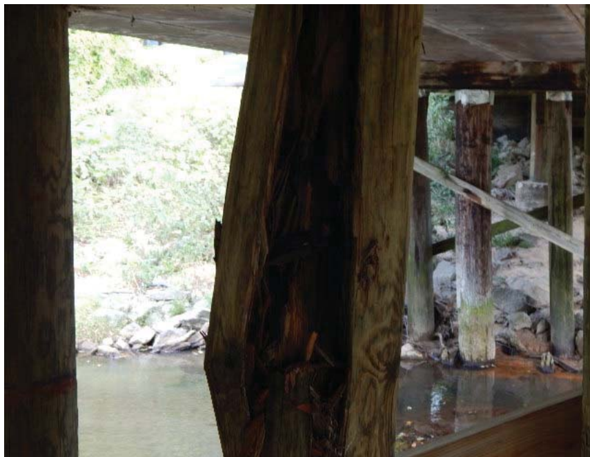
BENT 1 A PILE "C"
