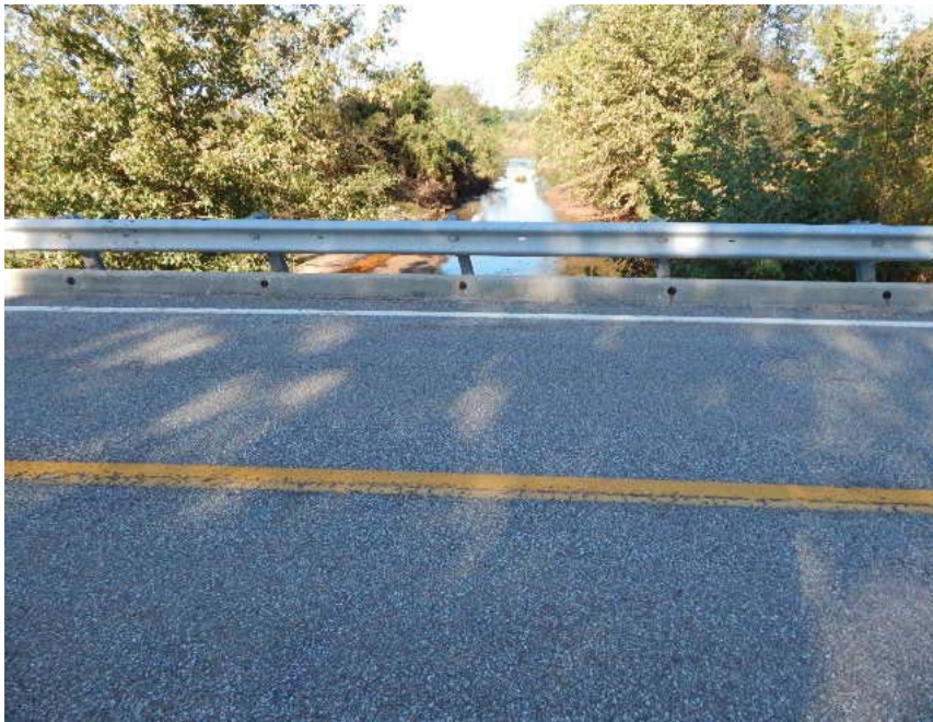
VIEW ACROSS TOP OF DECK
