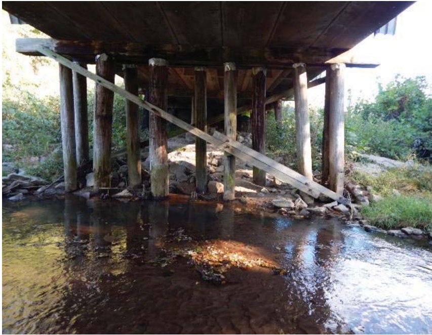
BENT 2 FRONT SIDE
