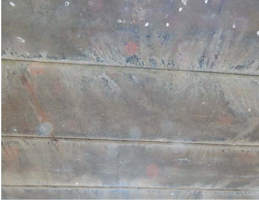
SPAN 2 BOTTOM DECK
