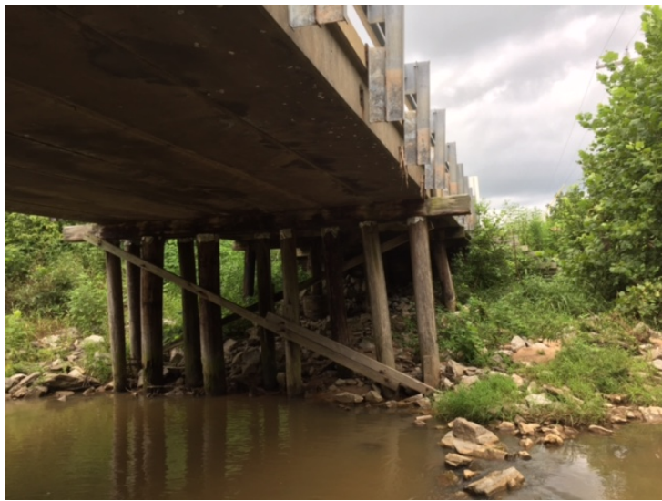
Photo 4. WWC-1/Looking up drainage
